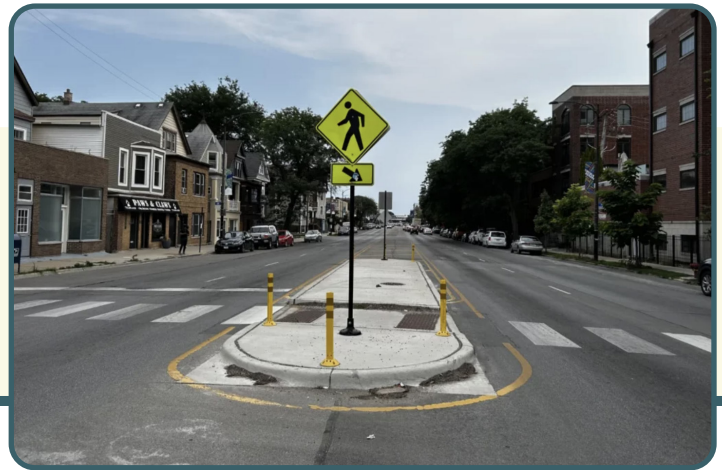
Installation of pedestrian island at Western/Winnemac through PB funding
