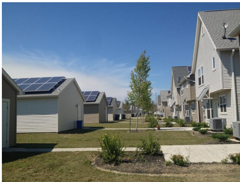
Figure 11 The Heritage View Homes were built to Enterprise Green standards and include permeable pavement and solar electric panels on some garages.
