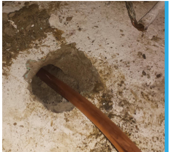
Figure 3. Trenchless pipe replacement – inside house, pulling new service line out of building
