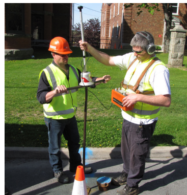
HALIFAX WATER STAFF INVOLVED IN LEAK DETECTION ACTIVITIES
